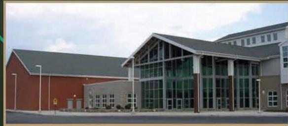
The student commons entrance is shielded by a triple-glazed curtain wall system (0.16 U-value). The commons ceiling uses tongue and groove planking from sustainable harvested wood.
