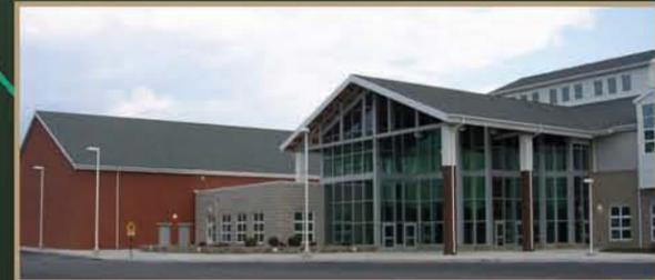
The student commons entrance is shielded by a triple-glazed curtain wall system (0.16 U-value). The commons ceiling uses tongue and groove planking from sustainable harvested wood.
